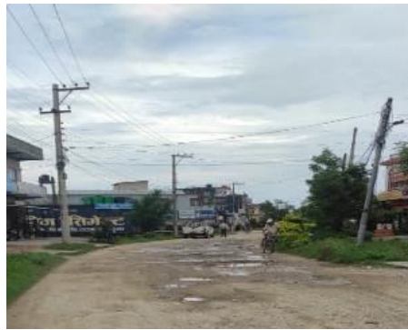
Existing condition of the road
