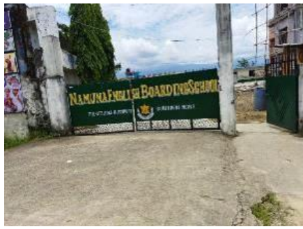
School gate and fence adjacent to RoW of road
