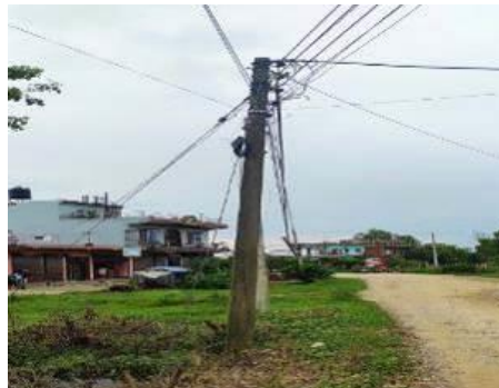
Electric Poles within the RoW to be relocated
