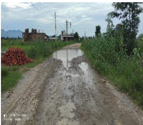
Physical condition of the road
