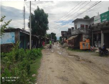
Tree within the RoW to be removed
