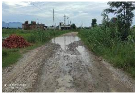
Condition of existing road
