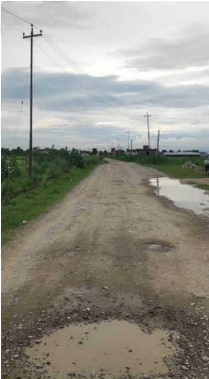
Condition of existing road
