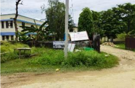
Pole at RoW
