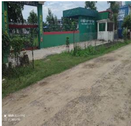
Condition of existing road
