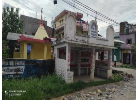
Public waiting place along the road alignment in Ward 7
