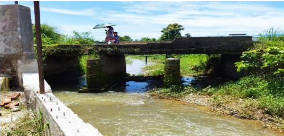
Bridge near Tilottama-7 ward office
