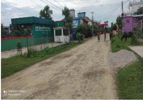
Condition of the road in Ward on 7
