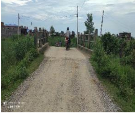
Bridge Structure at RoW
