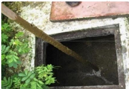
Checking sludge levels
