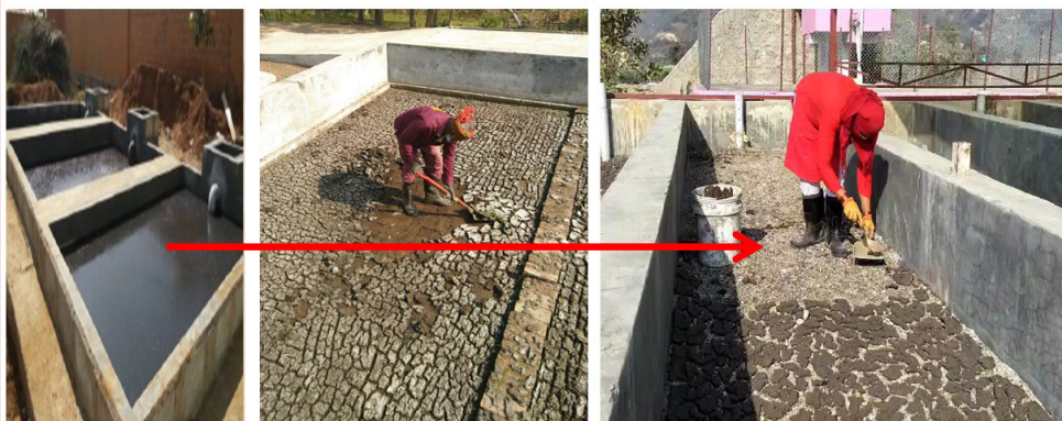
Example of the unplanted sludge drying bed
