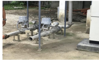
Pneumatic Valve Arrangement at Mechanized FSTP
