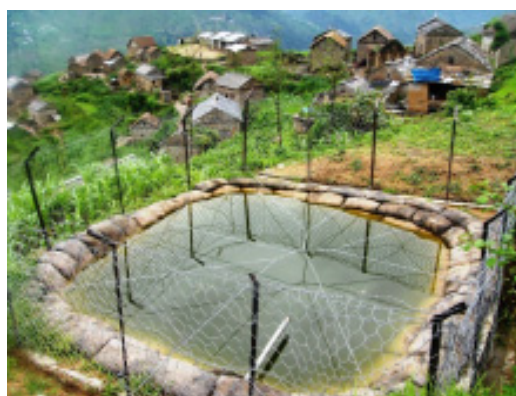
Figure 3: Pond with soil cement jute bag lining
