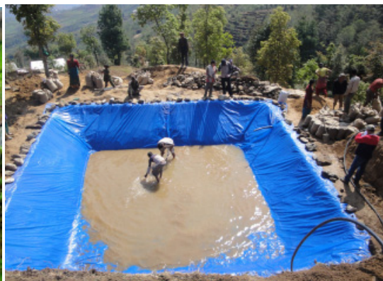
Figure 2: Excavated Pond with Lined
