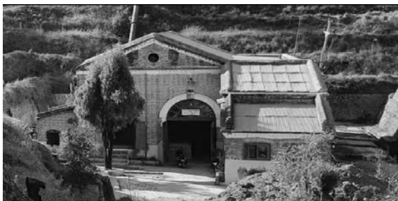
Figure 6 Pharping Hydropower Station ( https://en.wikipedia.org/ )
