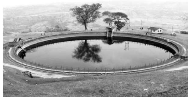
Figure 7 Pharping Hydropower Station ( https://en.wikipedia.org/ )
