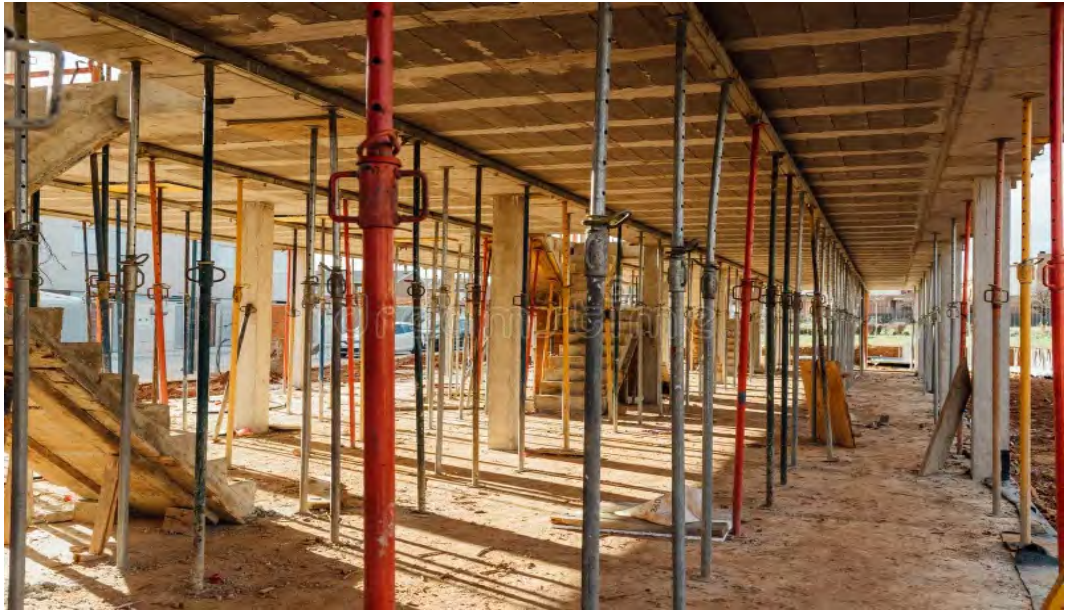
Figure 27 : Props and shuttering
