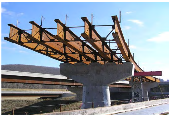
[Fig.10.1 Girders of suspension bridge]
