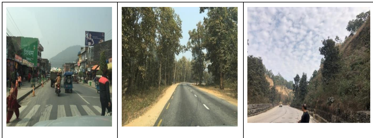
Figure 1: Existing Road Condition of Pathalaiya-Hetauda-Narayanghat (PHN) Road
