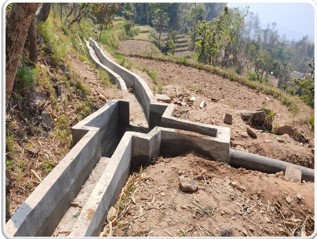
RCC canal lining & Division Box
