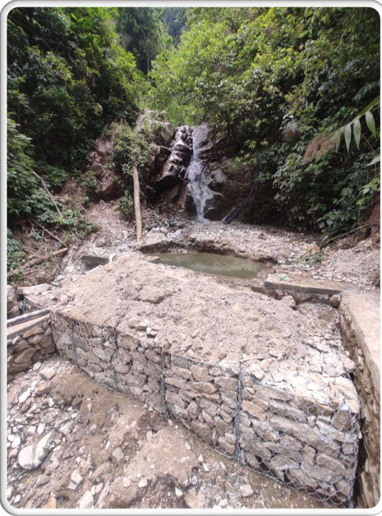
Intake at Gyami khola, Collection Chamber and Pipeline works.
