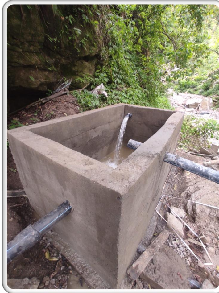
Intake at Gyami khola, Collection Chamber and Pipeline works.
