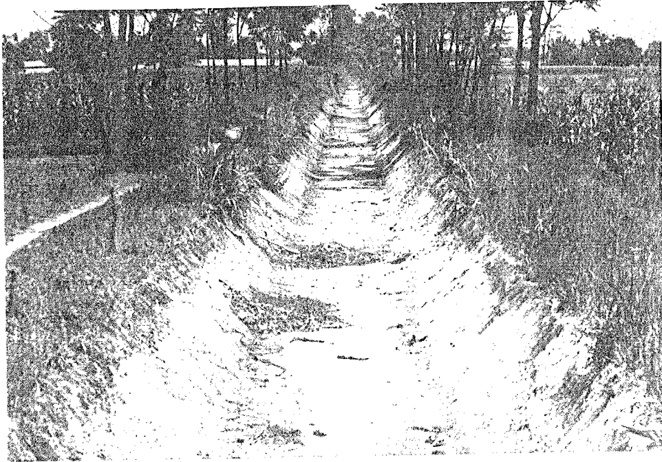
Photo – 22: Cleaned section of lined canal (branch – 6) Khageri Irrigation System
