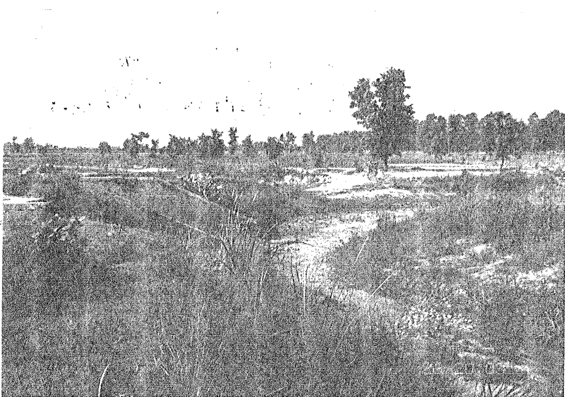
Photo – 29: Drain damaging Bishnuganj branch Nepal West Gandak Irrigation System
