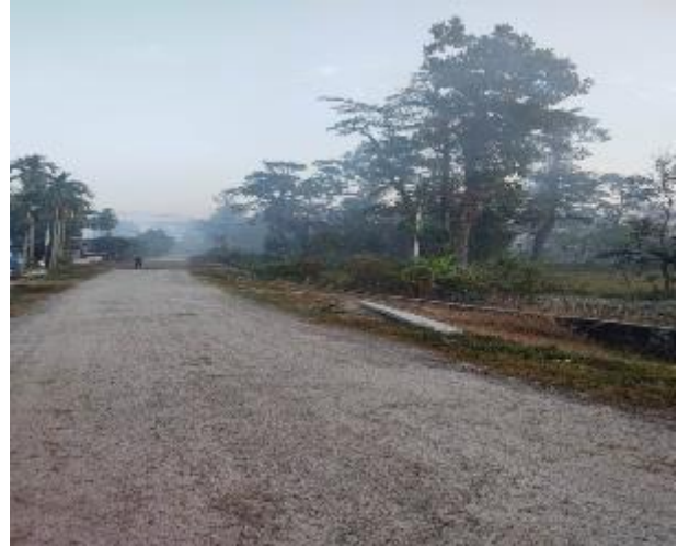
Road condition Ch 0+000 toward Gol chowk
