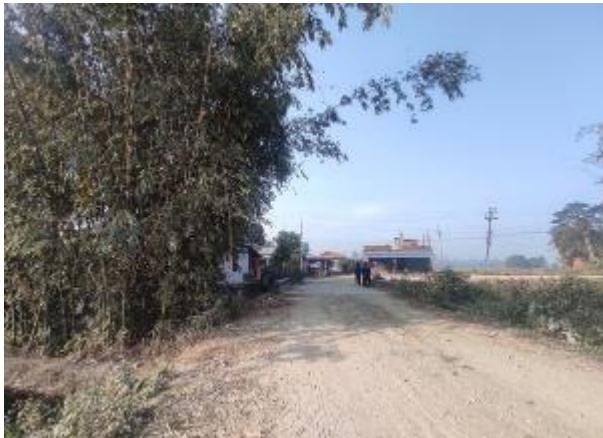
Road condition Ch 0+633 to 1+100, Saalbari
