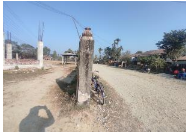
School wall within a ROW at Ch 2+080
