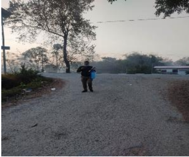
Starting point joining E/W Highway
