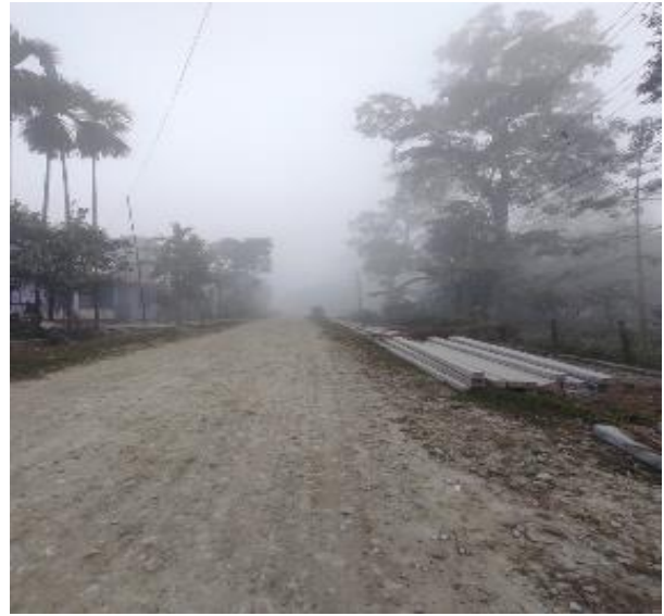
Existing condition of the road
