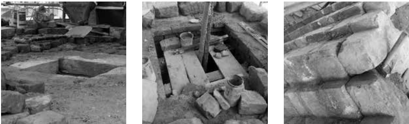
Figure 5- Pictures at time of restoration, from left-central hole of first floor, main body of Shikhara showing masonry, outer face of Shikhara.
