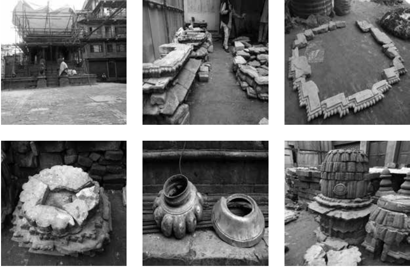
Figure 3- Pictures showing the storage of dismantled elements of temple as per munbering done.
