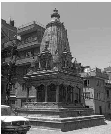
Figure 9- Temple after completion of restoration work.
