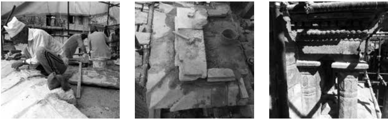
Figure 4- Pictures showing conservation works in different levels of cornices source authors.
