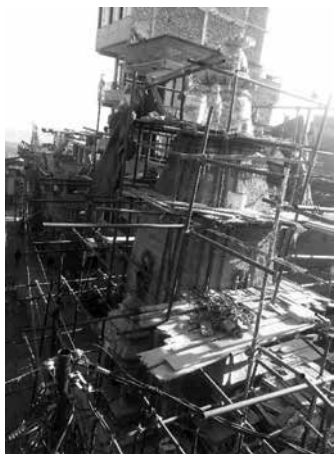
Figure 8- Temple during restoration work.
